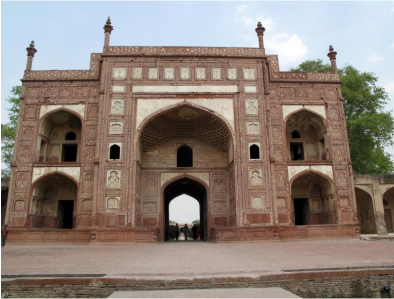
Figure 1 Jehangir mausoleum entry gate--all photos from 2009
